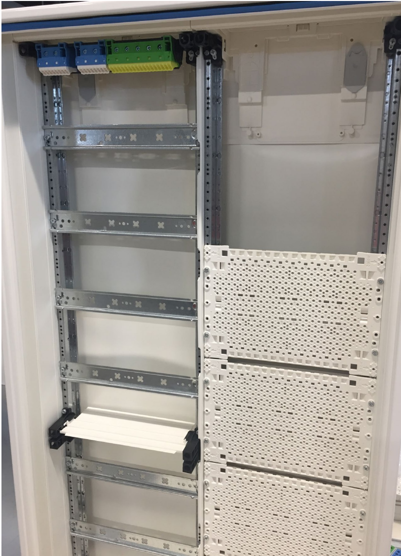
Cabinet with installed partitions
