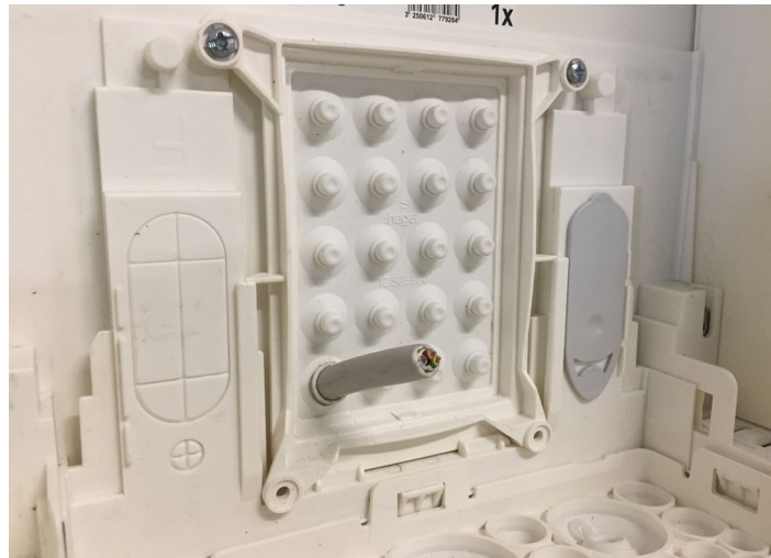
Flange FZ428 installed on the rear of the cabinet
