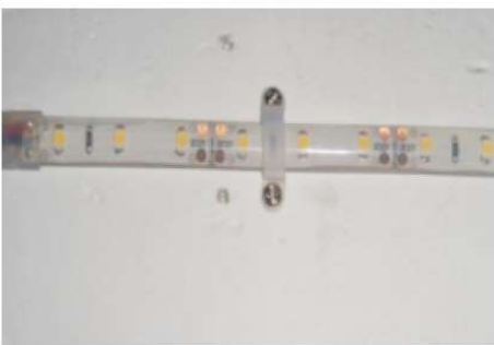
○ Installation is finished;
