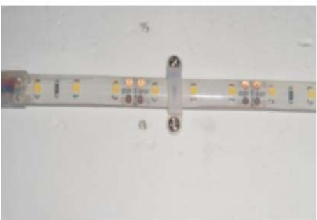
○ Installation is finished;
