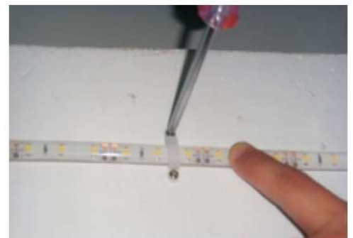
○ Install the snap spring;
